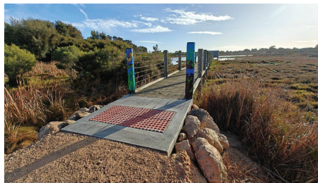
Pictured above: Construction of Meningie Wetlands Boardwalk access ramp now complete.
