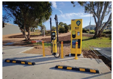
Pictured above: Post-concreting of RAA EV charging station, Meningie.
