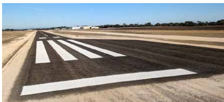
Pictured above: Tintinara Aerodrome after line marking.
