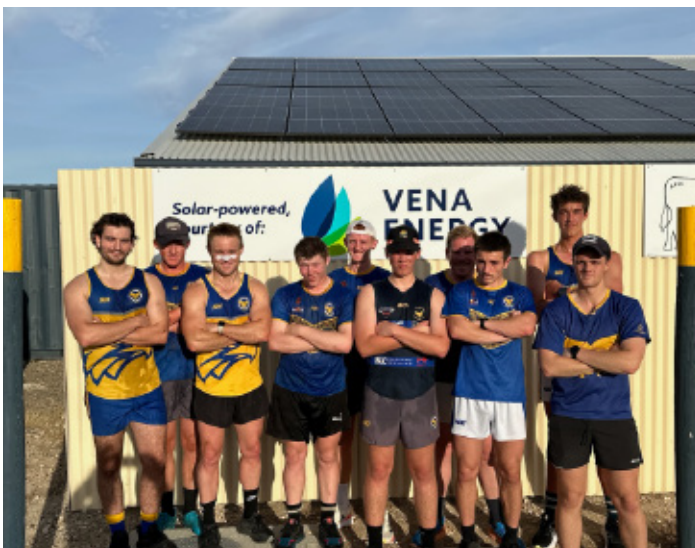
ABOVE: The Tailem Bend Football Club with new solar panels.
